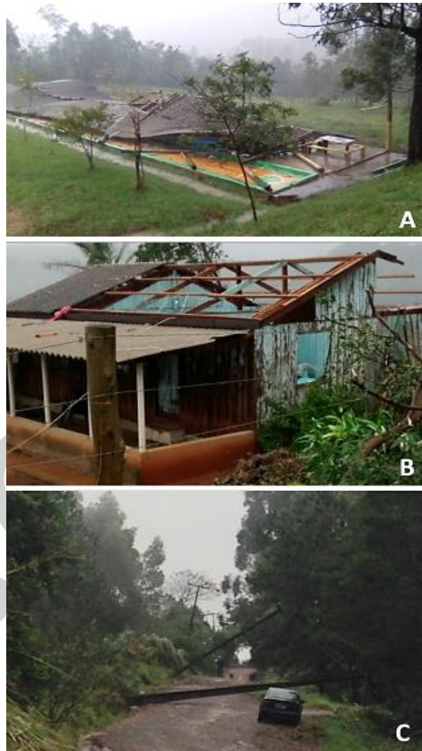
Fig. 3 Photos of damage caused by alleged Tornado in Rio Branco do Ivaí [3]. The destruction of property (A), home (B), and poles of the electric power grid (C) is clearly evident.
